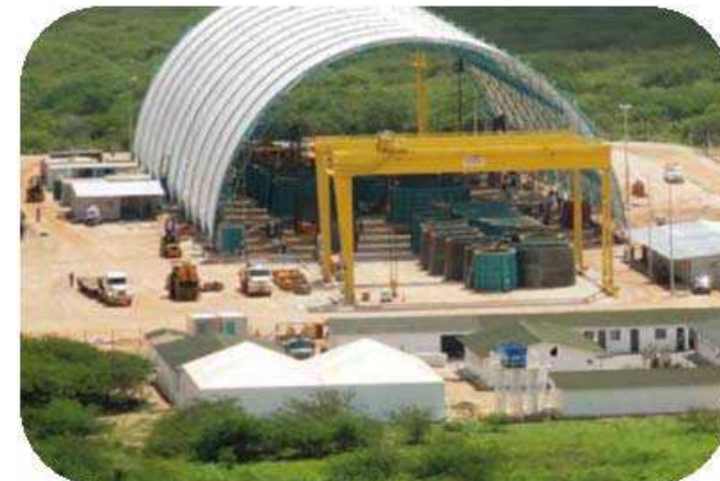
Concrete tower manufacturing site
