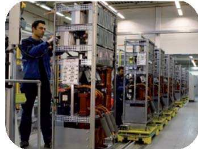
Power converter facility in Niagara (2012)
