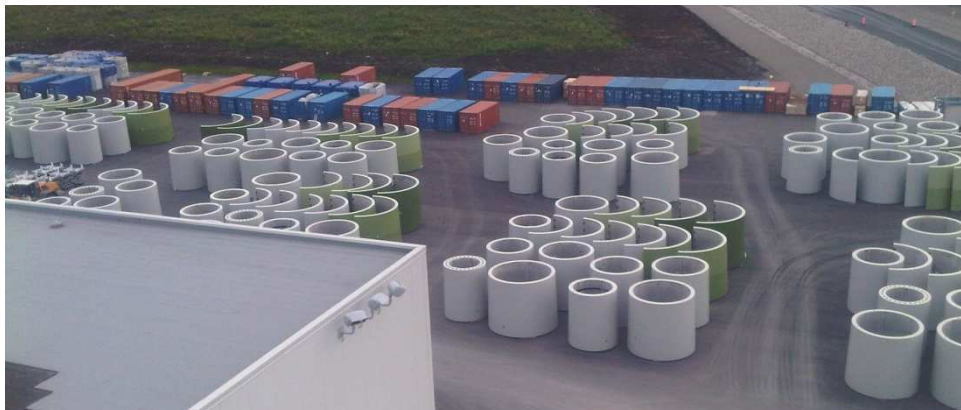
Serial production of pre-cast concrete towers
